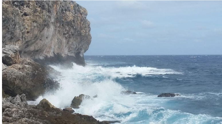
The Wave Wall getting battered by high seas. Arsenault
