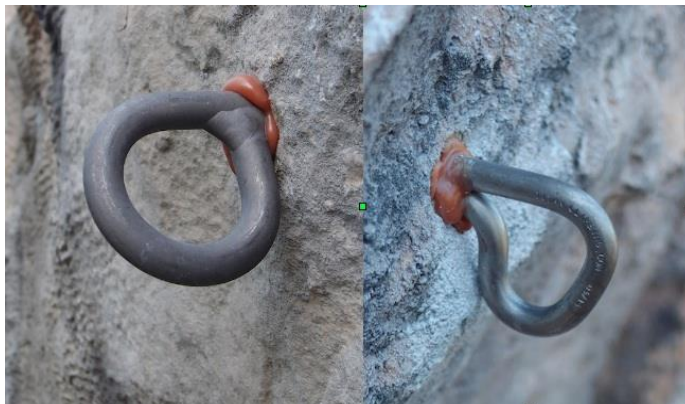
The 2 types of titanium bolts on Brac: round Tortuga bolt (left) & pear-shaped Eterna bolt (right)
